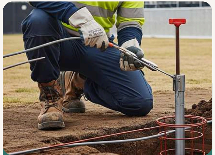
Connection: Connect cleaned conductor securely and apply anti-corrosion protection
