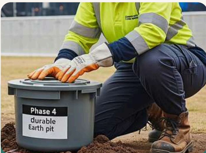
Backfilling: Backfill in layers and install labeled earth pit cover
